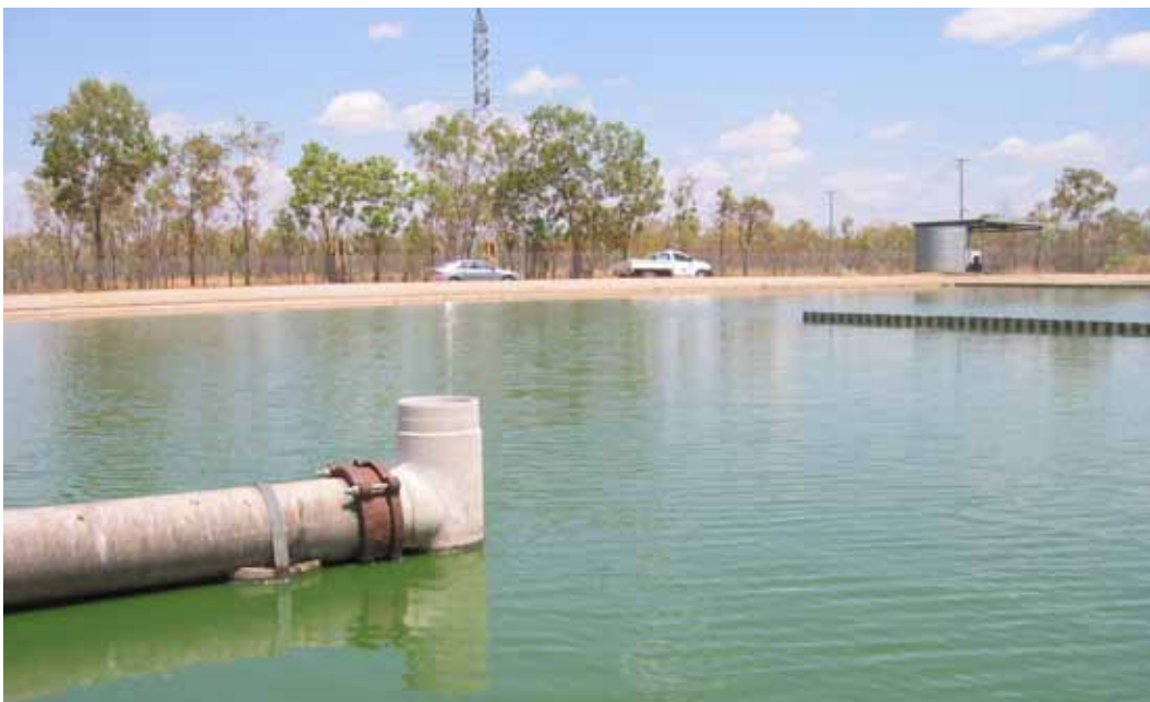
FIGURE 6.6 POND CURTAINING
