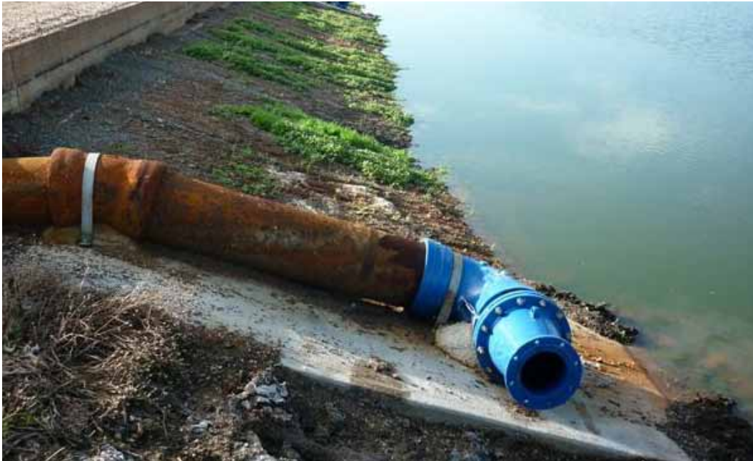
FIGURE 6.5B THE PREFERRED INLET PIPE NOZZLE AND DIRECTION
