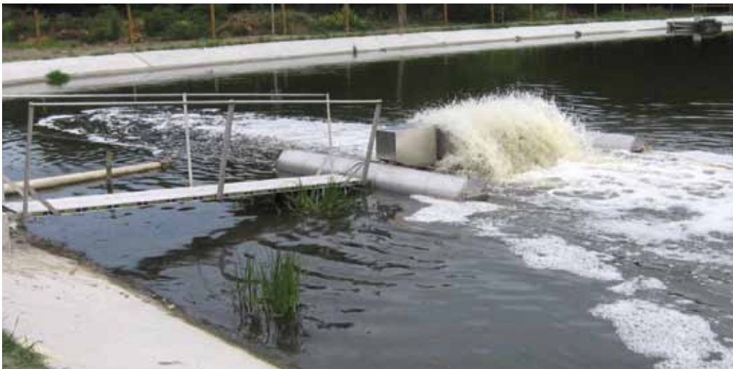
FIGURE 6.8 BRUSH MIXER AND AERATOR
