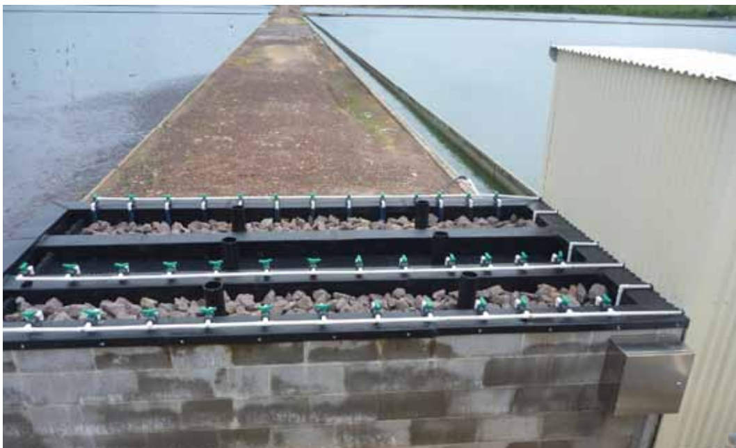
FIGURE 5.3 PILOT AERATED ROCK FILTER
