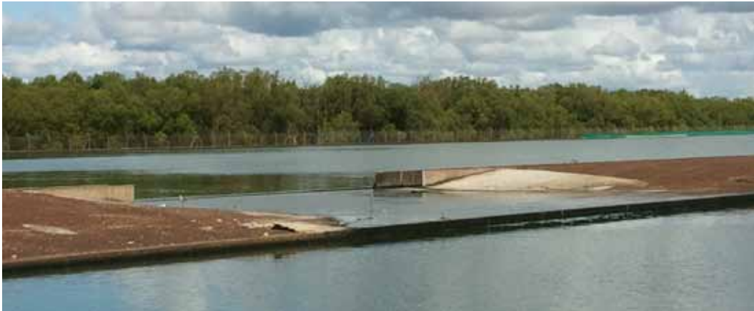
FIGURE 6.1 STORM OVERFLOW EMBANKMENT SPILLWAYS BETWEEN TWO PONDS
