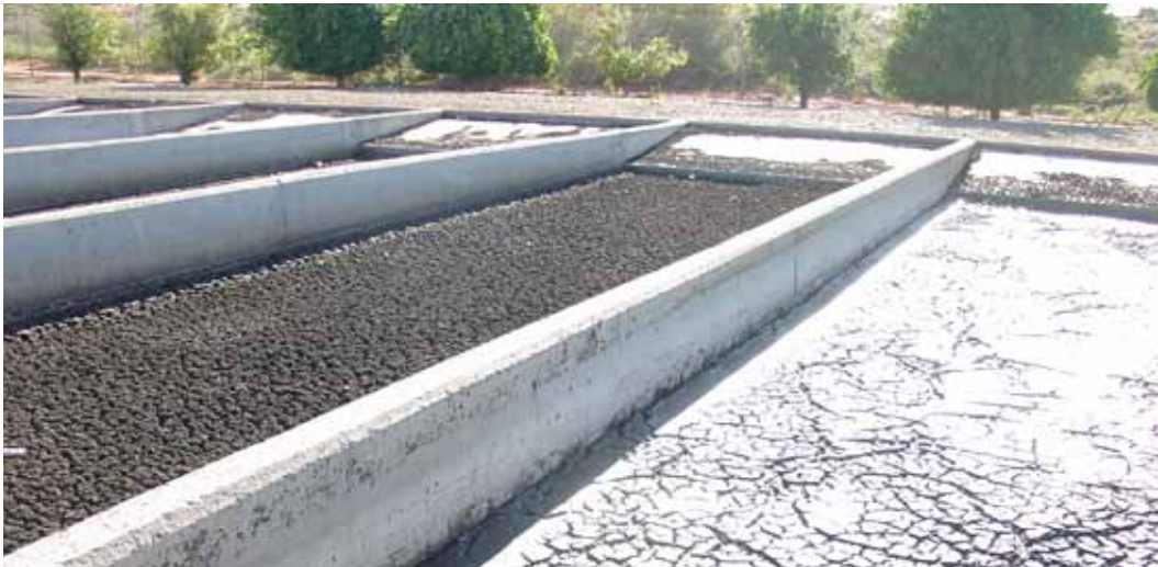
FIGURE 11.1 WSP SLUDGE DRYING BEDS
