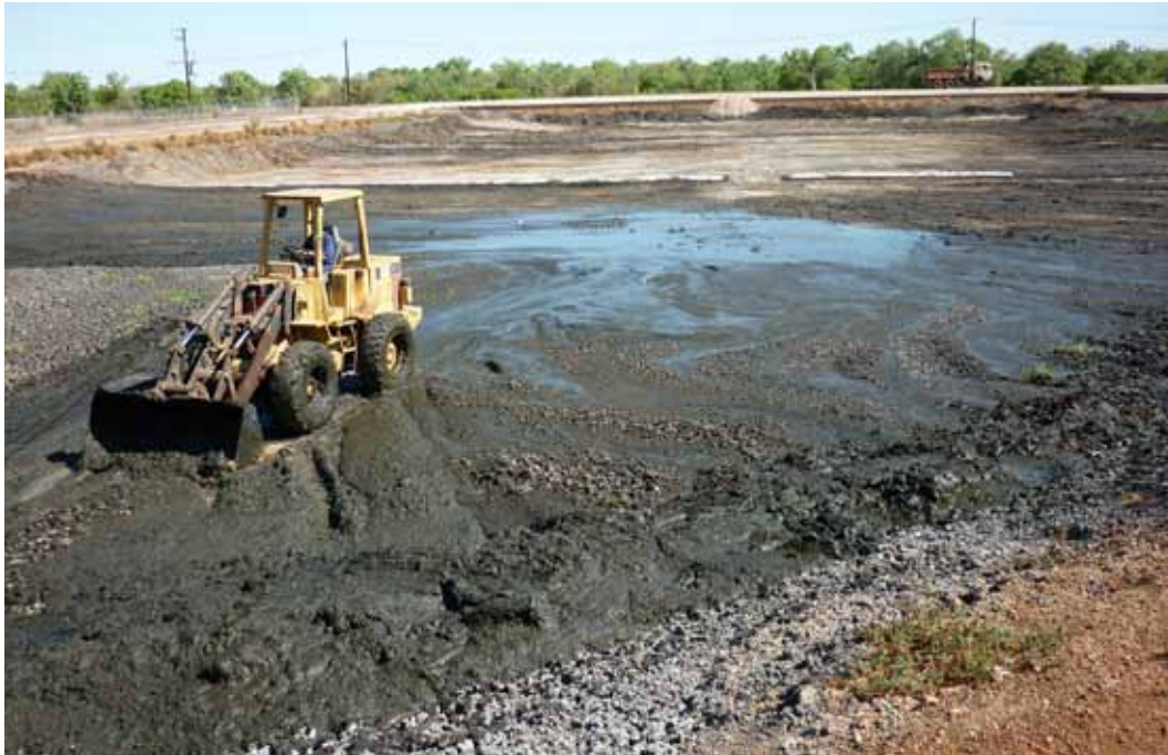
FIGURE 4.3B DESLUDGING THE POND ABOVE AT THE FINAL MOPPING UP STAGE
