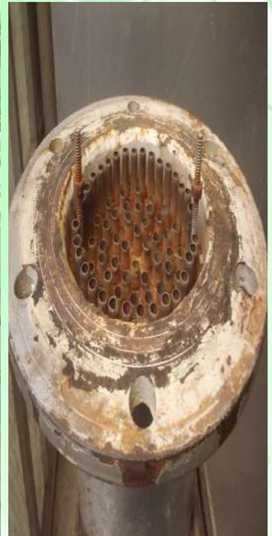
Liquid Redistribution unit in the new modified water scrubbing tower at IIT Delhi
