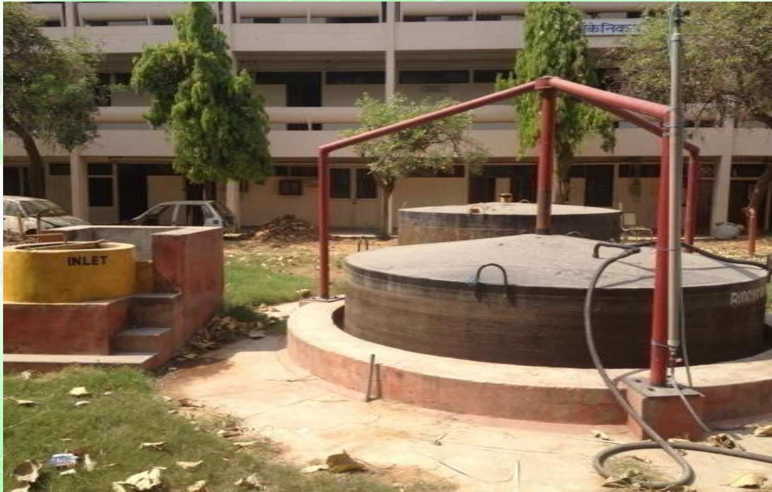
Biogas Plant at IIT Delhi
