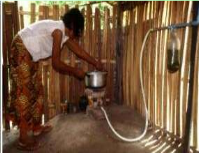
Pipeline for raw biogas use as a cooking fuel
