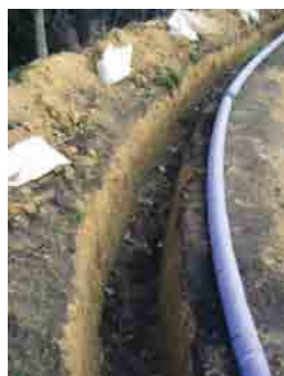
Perimeter trench and biogas transfer pipe:
