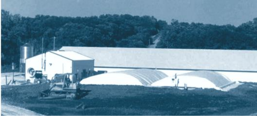
Figure 9 Photo of a Mixed Digester (EPA, 2002)
