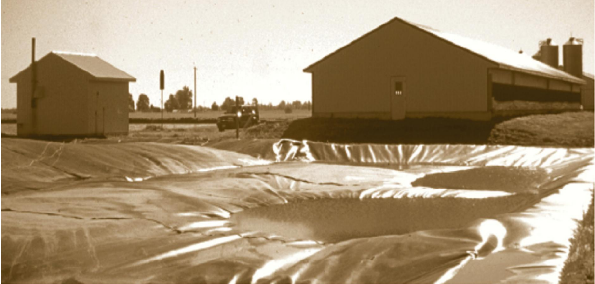
Figure 8 Photo of a Covered Anaerobic Lagoon (EPA, 2002)
