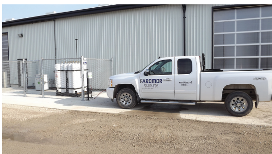
Photo: CNG Energy Group
