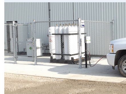
Photo: CNG Energy Group
