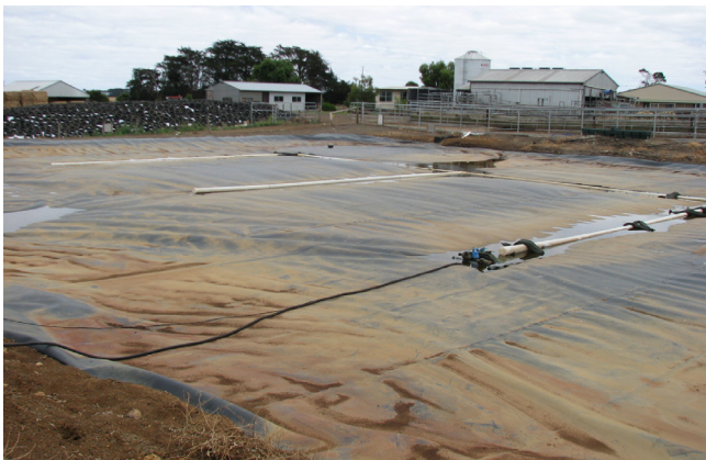
Covered anaerobic pond. Photo courtesy of DemoDAIRY
