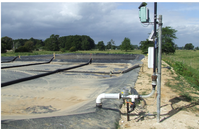
Covered anaerobic pond and candlestick flare. Photo courtesy of NIWA
