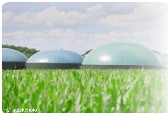
© istockphoto® Biogas storage containers
