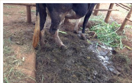
Cement stall flooring in poor condition making manure and urine collection difficult
